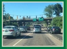
The current interchange at Exit 16 is a grade separated tight diamond interchange with I-89 crossing over U.S. 2/7 via two bridges. The existing interchange yields frequent traffic congestion, lengthy delays, and significant queuing during peak hours. These existing conditions are a safety concern with a high number of incidents, collisions, and a lack of accommodations for non-motorized travel.
